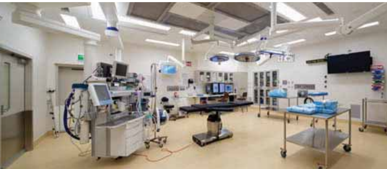
Figure 2: Orthopaedic operating theatre, Townsville Hospital, Queensland: The impact of equipment and technology on human factors is not discussed early in the design process
