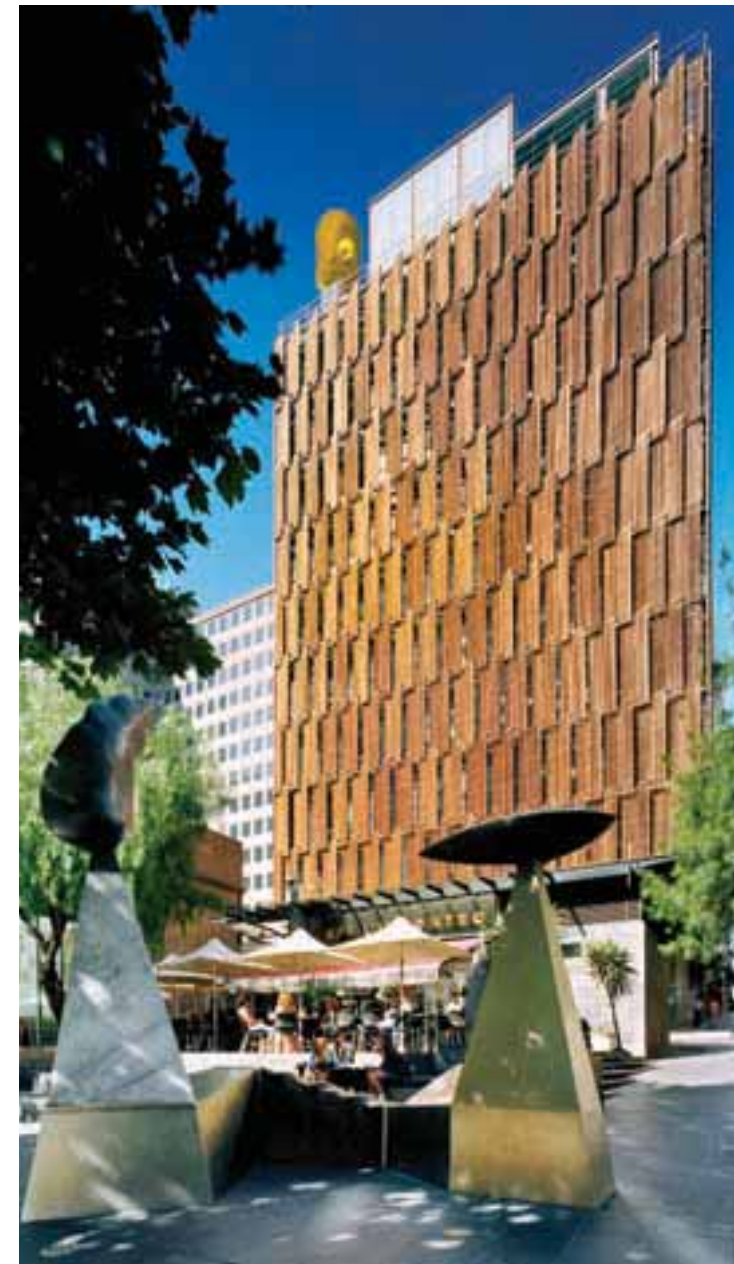
Figure 3: DesignInc's Council House 2, which is owned and occupied by the City of Melbourne, was the first office building in Australia to receive a six-star rating
