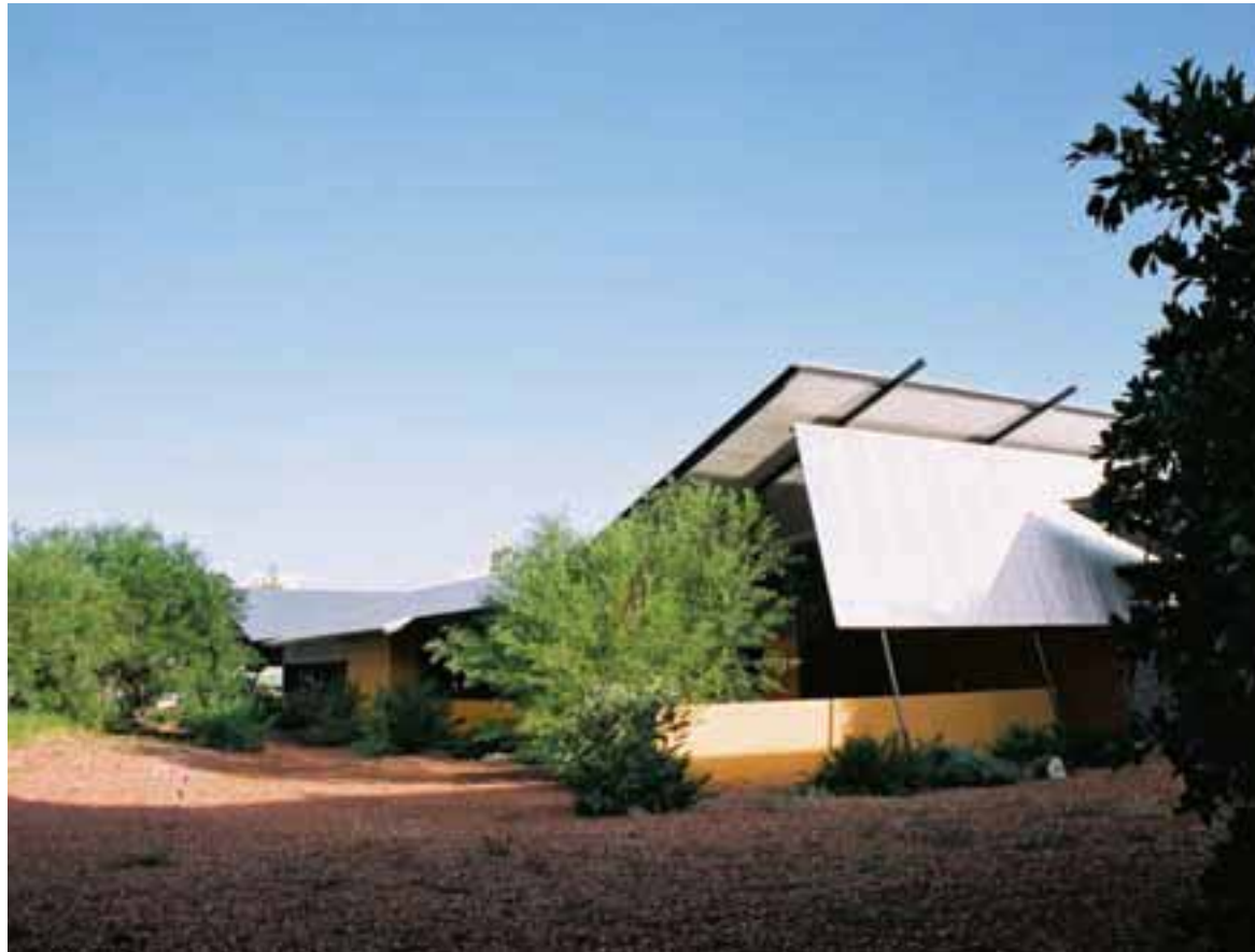
Figure 5: Tennant Creek renal clinic combines a hi-tech fit-out with a friendly external appearance, using scale, materials and landscaping
