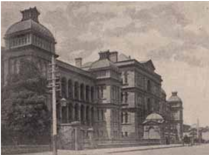
Figure 2: Sydney Hospital, the oldest hospital in Australia, opened in 1816. The building almost immediately had to be extensively repaired, due to its poor-quality construction
