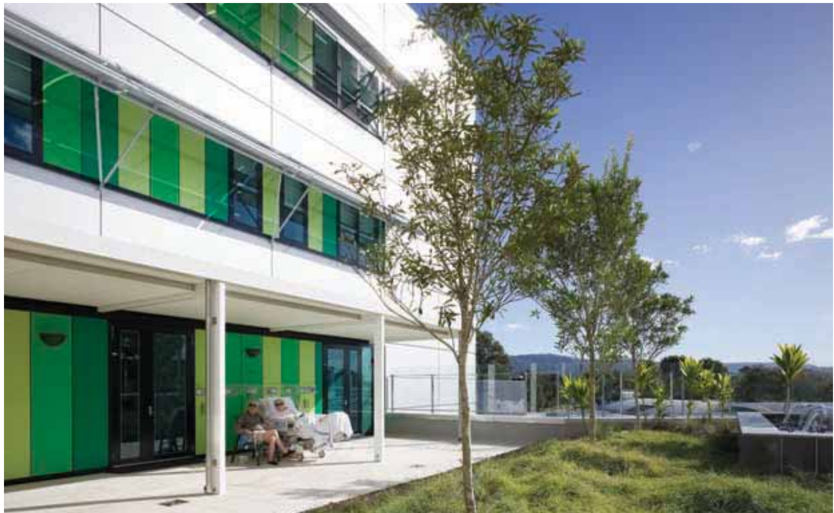
Figure 3: At BVN Donovan Hill's Robina Hospital, beds for palliative care patients can be moved outside – just one result of a more people-focused approach
