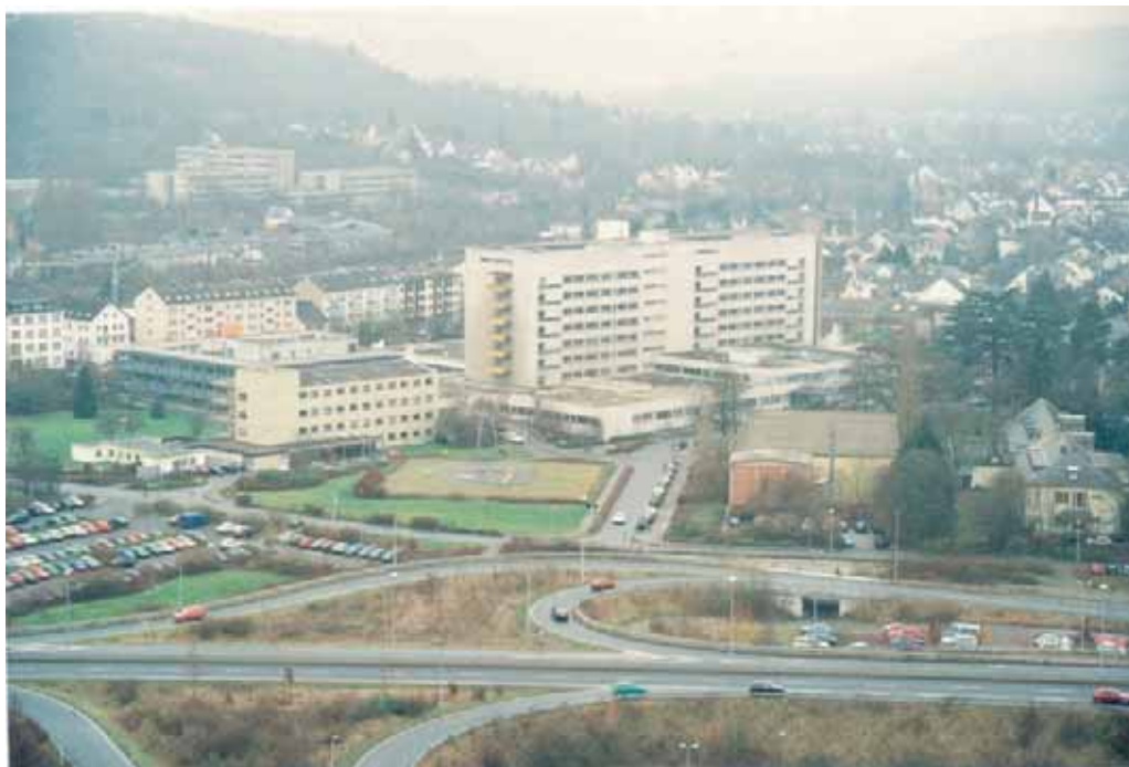
Figure 1 View of the Kemperhof Hospital in Koblenz/ Germany
