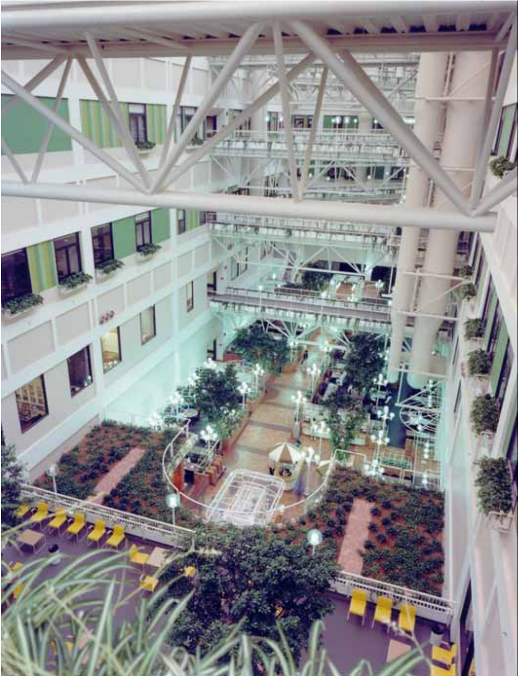
Figure 5 Walter C. Mackenzie Health Sciences Centre, Edmonton, Alberta, Canada
