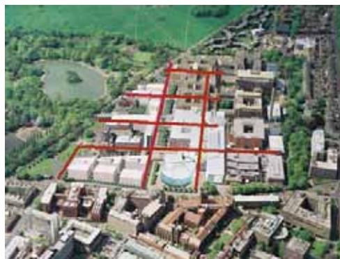
Figure 1 Red lines indicate major hospital circulation routes. Left-hand vertical line represents external mall. Right-hand vertical line represent internal gallery
