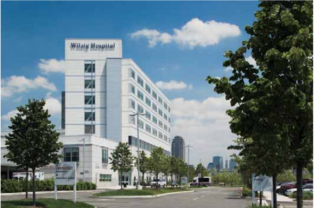
Figure 14 Jersey City Medical Center Exterior View
