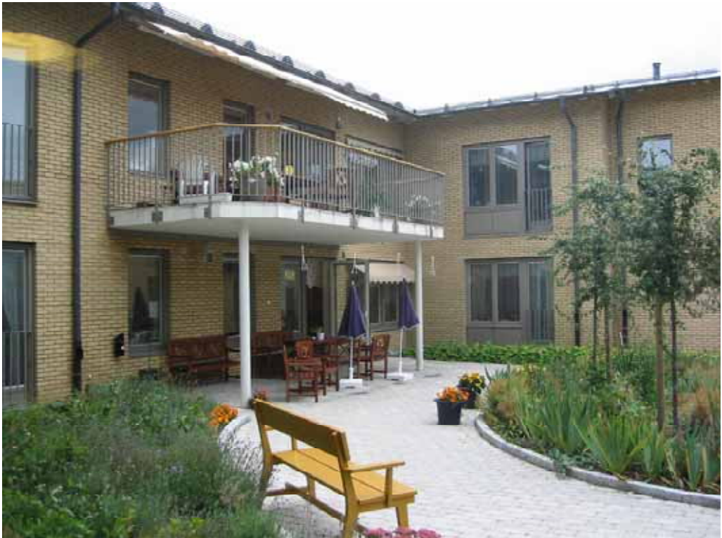
Figure 1 Balcony and seating outdoors
