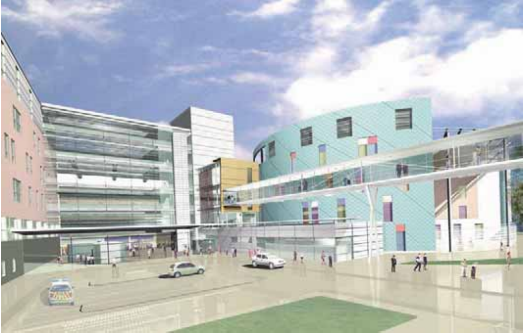
Figure 3 View of the main entrance with distinctive copperclad drum of Children's Hospital to the right.
