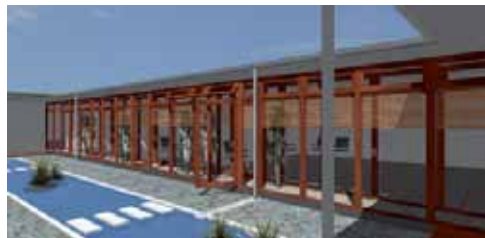
Figure 2 The building envelope of the new hospital uilding at Fachkrankenhaus Nordfriesland has been designed with high insulation levels and a double skin façade. Windows are optimized for additional ventilation, daylighting and visual comfort.
