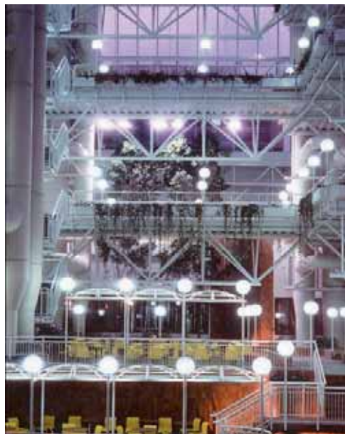
Figure 4 Walter C. Mackenzie Health Sciences Centre, Edmonton, Alberta, Canada
