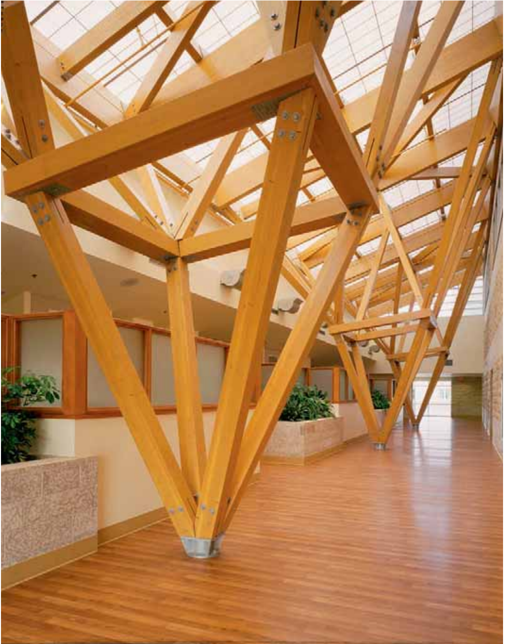
Figure 6 Wood trusses mark the entry to cancer treatment bunkers
