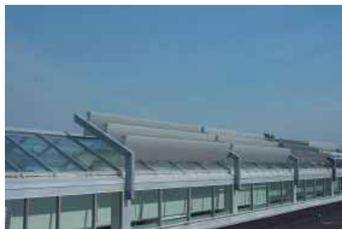
Figure 5 Shading devices at Aabenraa Hospital.
