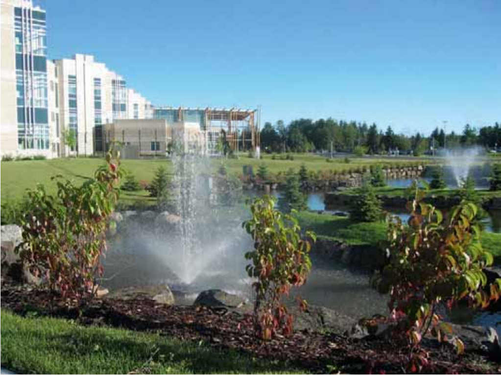
Figure 3 On-site stormwater retention ponds cleanse rainwater and provide fish habitats
