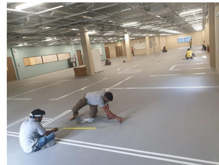
Taping and Placement of Walls On-site
