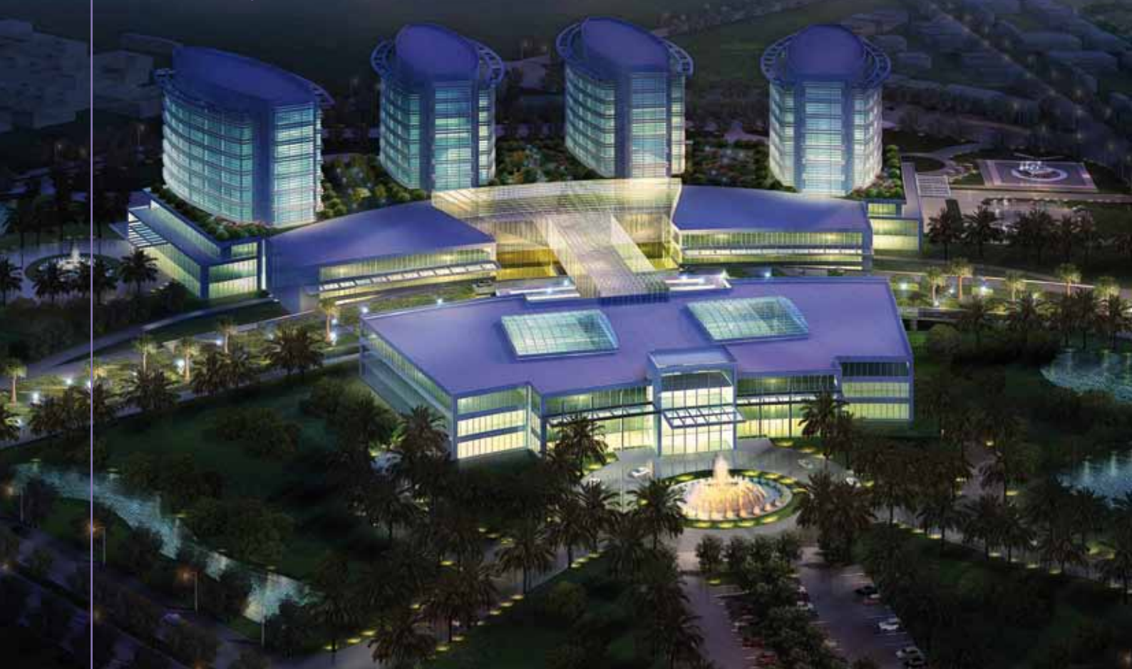
Above: Al Mafraq Hospital in Abu Dhabi, masterplanned for SEHA by Burt Hill
