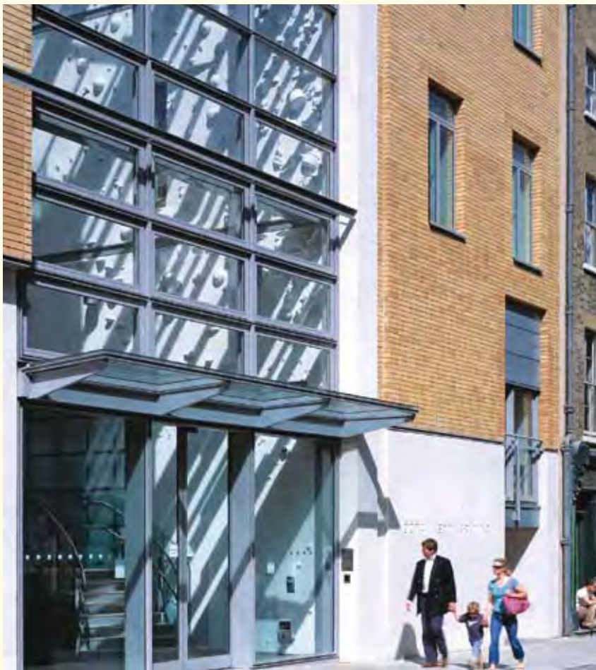
Anshen + Allen's Great Ormond Street Hospital, London: asthma is the leading cause of child hospitalisation
