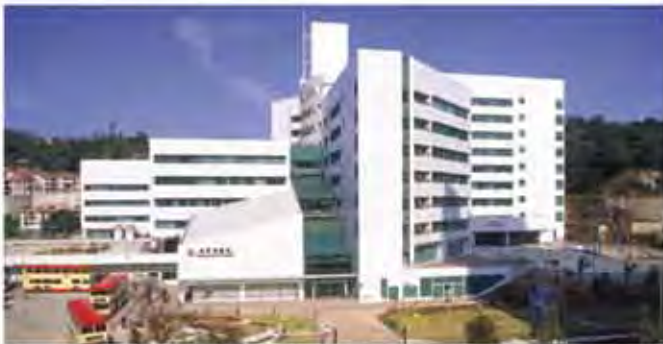
Tseung Kwan O Hospital, Hong Kong, China
