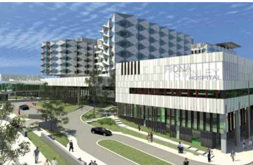
Fiona Stanley Hospital in Western Australia: a model for flexible, future-proof health facilities
