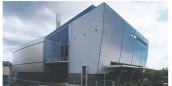
Princess Alexandra Hospital, Brisbane, Australia
