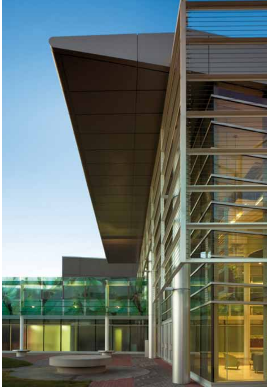
The Perkins Eastman Black-designed Trillium Health Centre in West Toronto was transformed into a garden of wellness, planned around a time-tested urban element: the street
