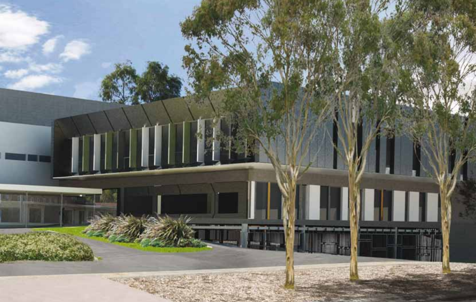
Currently on site, Nepean Hospital in Sydney's western suburbs will deliver extra beds and operating theatres
