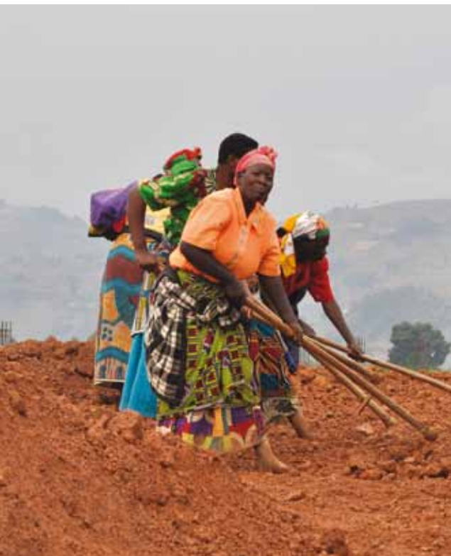
Rwanda's Butaro hospital was built entirely by a local workforce
