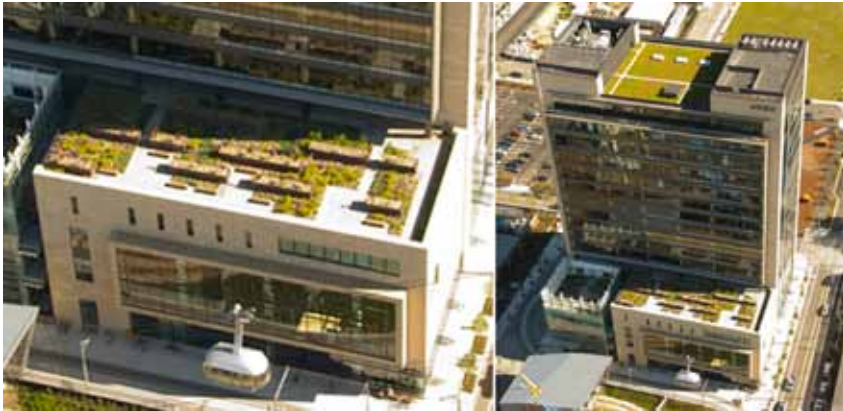
Figure 11: OHSU-CHH north and south green roof and cool roof
