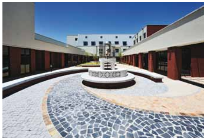
With much daily activity in the townships taking place outdoors, ACG incorporated many outdoor areas, including covered waiting areas, to create a sense of familiarity
