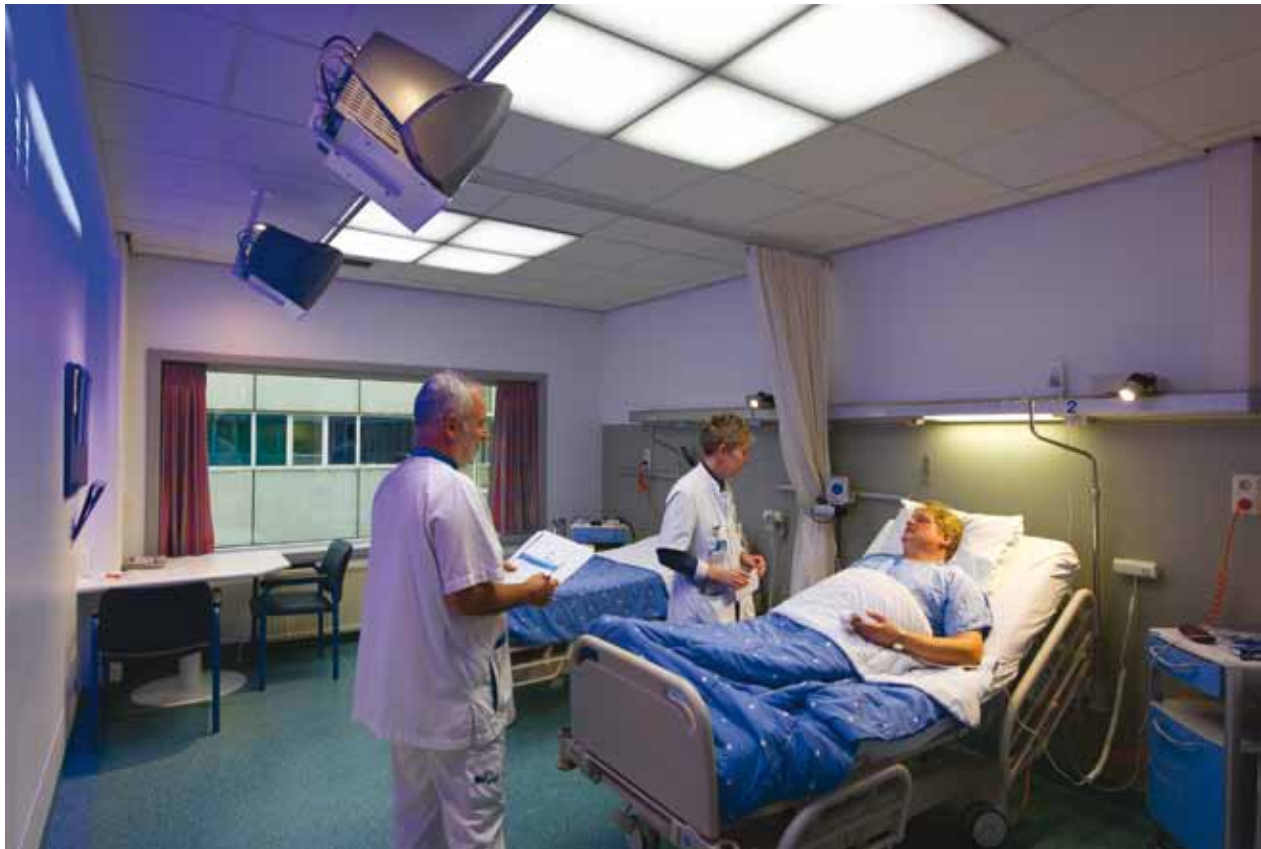
Tested at Maastricht University, HealWell (above) mimics daylight, helping to regulate patients’ body clocks and improve sleep. Top: a patient room without HealWell
