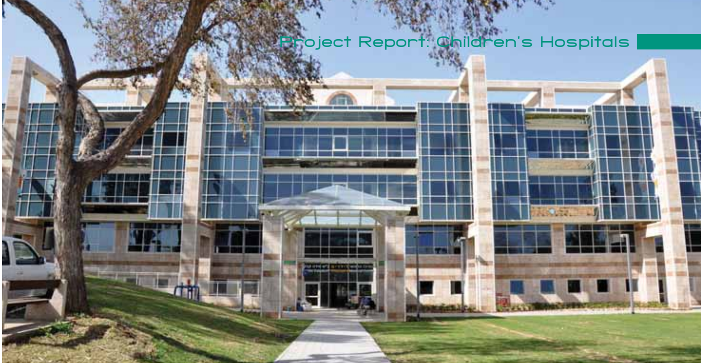
Israel's new children's medical centre replaces a series of 1950s barracks
