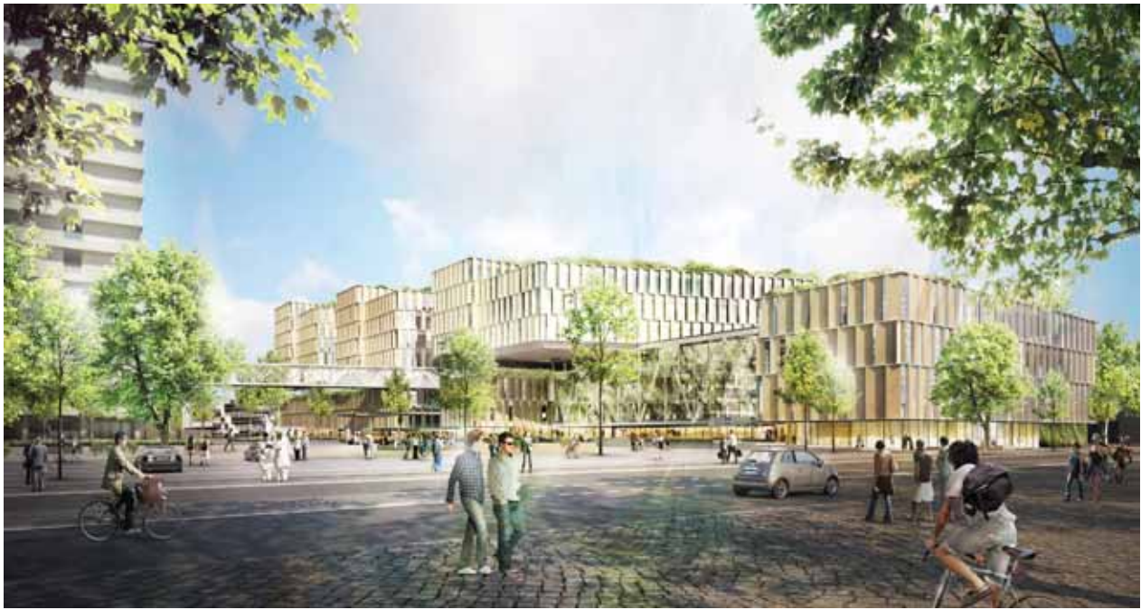
Copenhagen's main hospital is on a central urban site, but architects 3XN envisage a very green new extension
