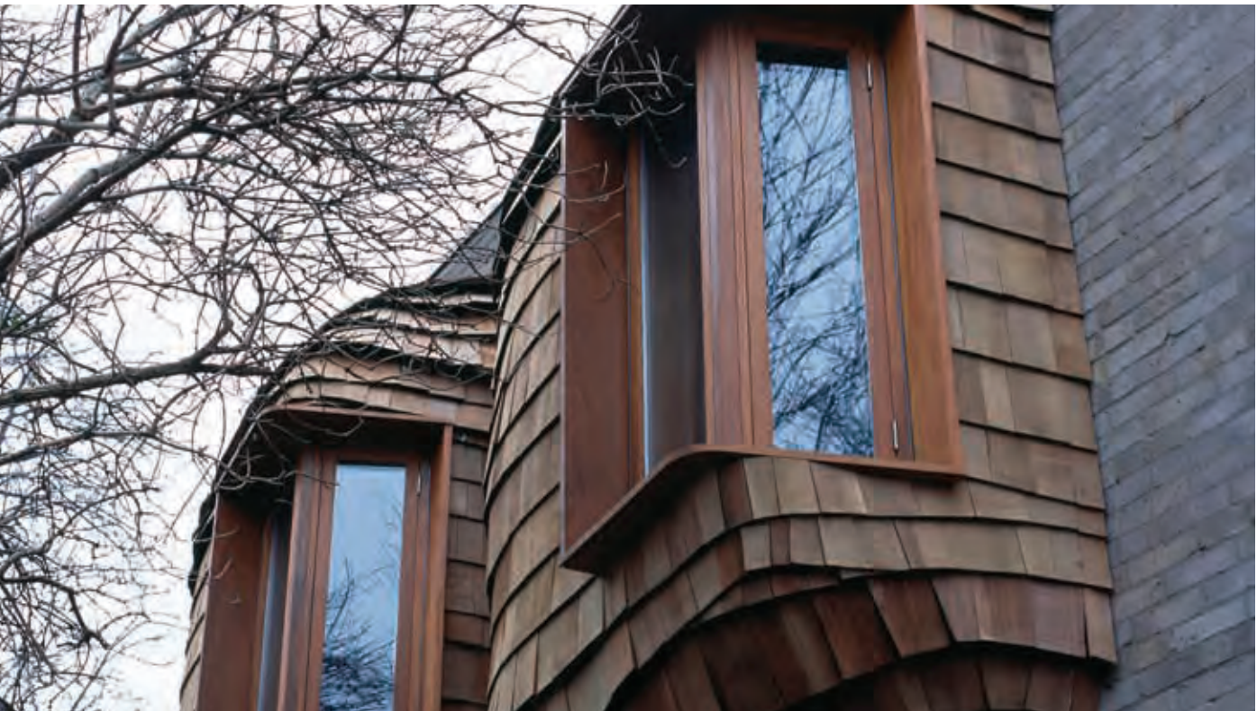
The South Essex Rape and Incest Crisis Centre (SERICC): Featherstone Young Architects' shingle-clad 'pods' help soften the building's external appearance
