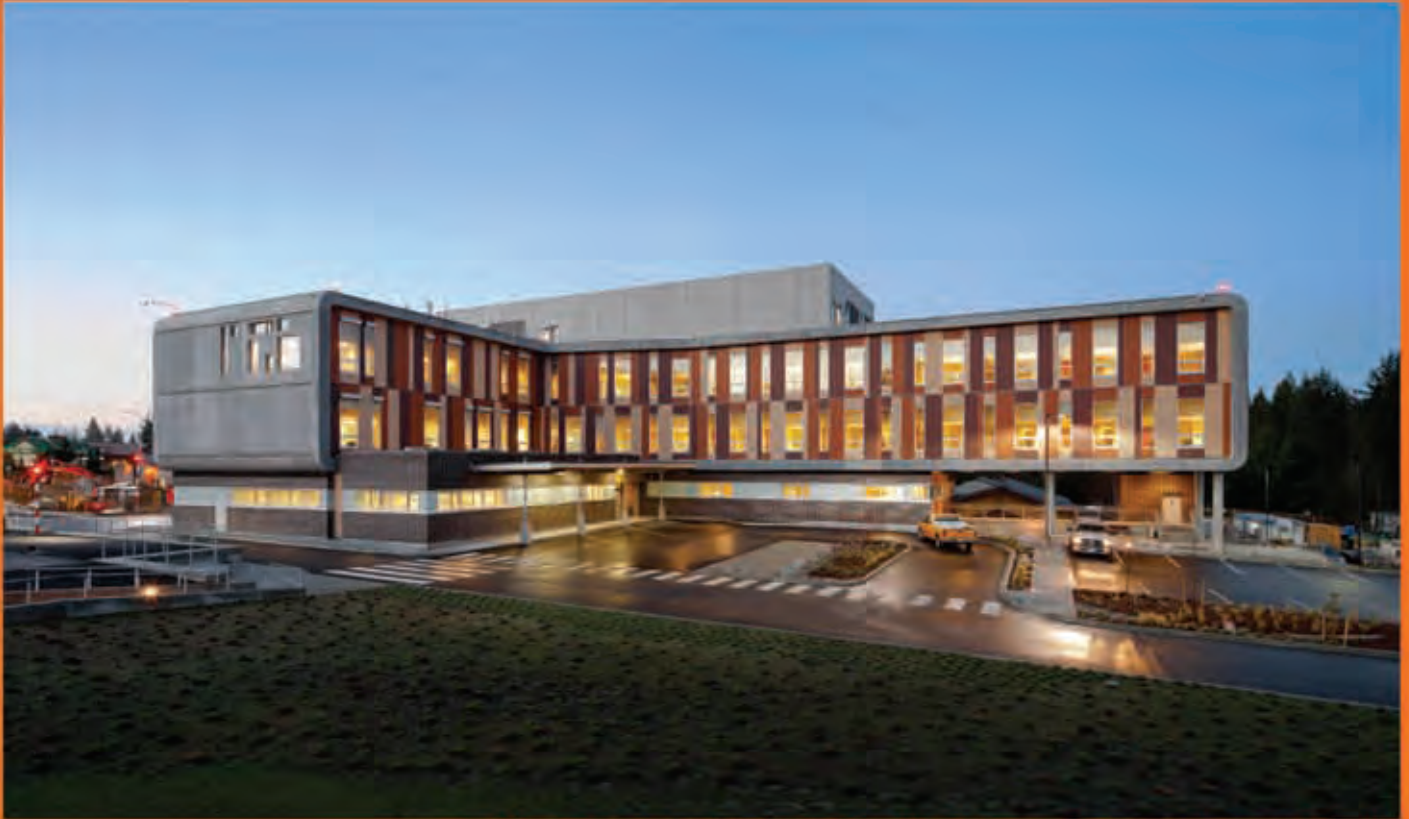
St. Mary's Hospital, Sechelt, British Columbia, Canada / Farrow Partnership Architects in association with Perkins+Will Image: Lafreille Delage Photography
