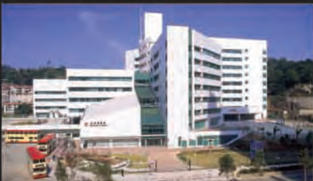
Tseung Kwan O Hospital, Hong Kong, China
