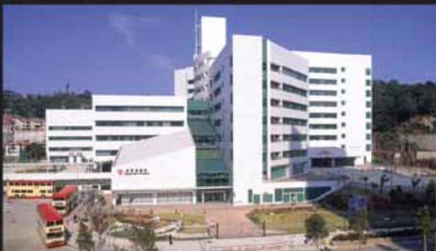
Tseung Kwan O Hospital, Hong Kong, China
