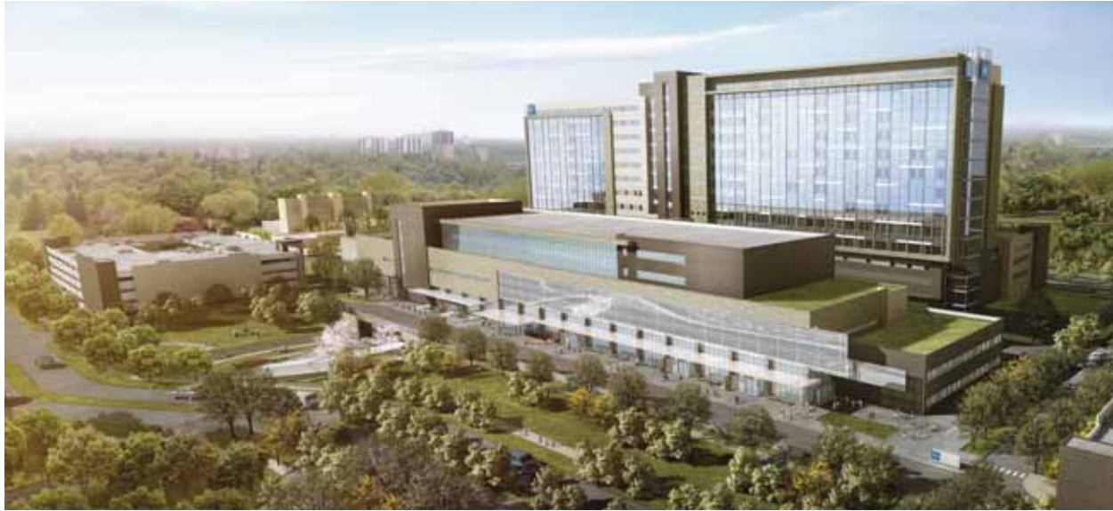
Humber River Hospital, Canada, designed by HDR
