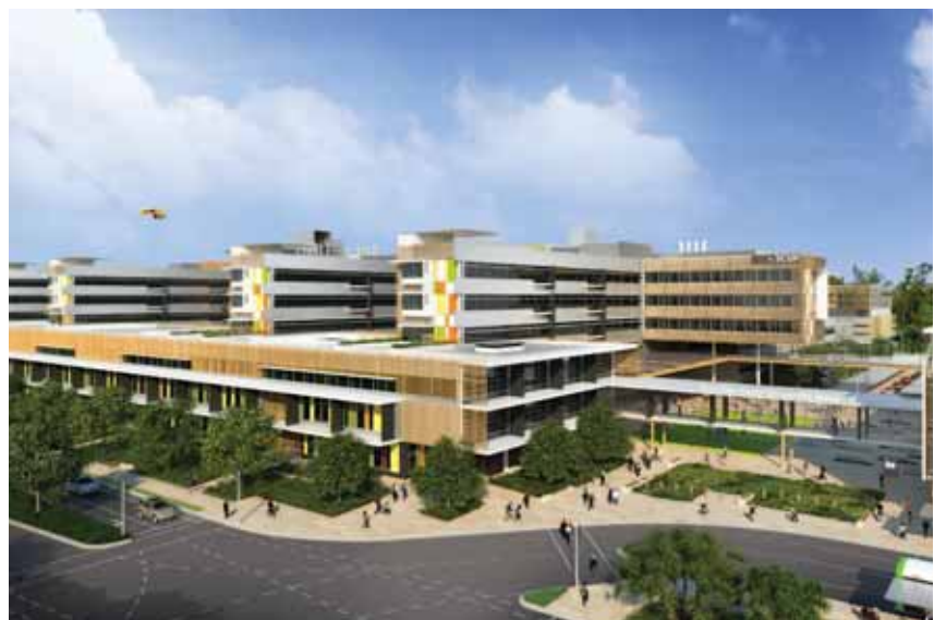
Public-private partnership: Sunshine Coast Public University Hospital, Queensland
