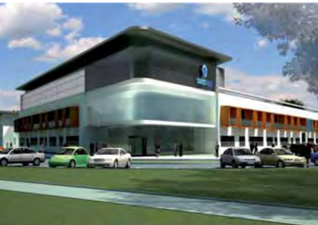
The WGI-designed Swissmed hospital in Warsaw, currently under construction
