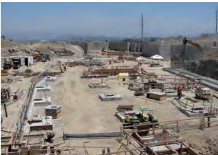
Palomar Pomerado Health's new hospital on site and under construction
