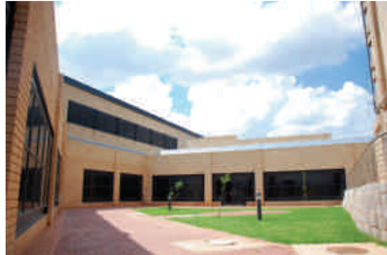
Figure 1.1: Chris Hani Baragwanath Hospital Main Internal Courtyard
