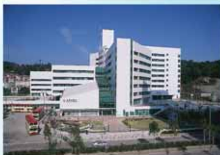
Tseung Kwan O Hospital, Hong Kong, China
