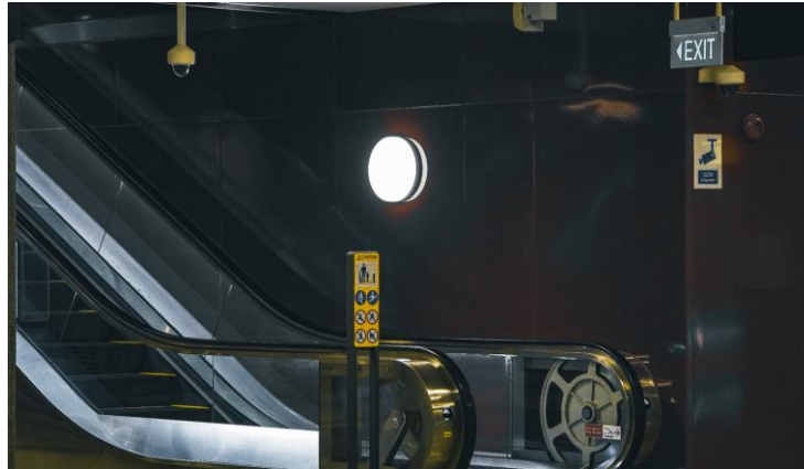
Lights at Orchard Station Exit 4
