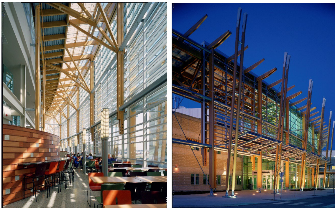
Images 12 & 13. The Thunder Bay Regional Health Sciences Centre. Salter Farrow Pilon Architects, of which Farrow Partners Architects is a successor firm.
