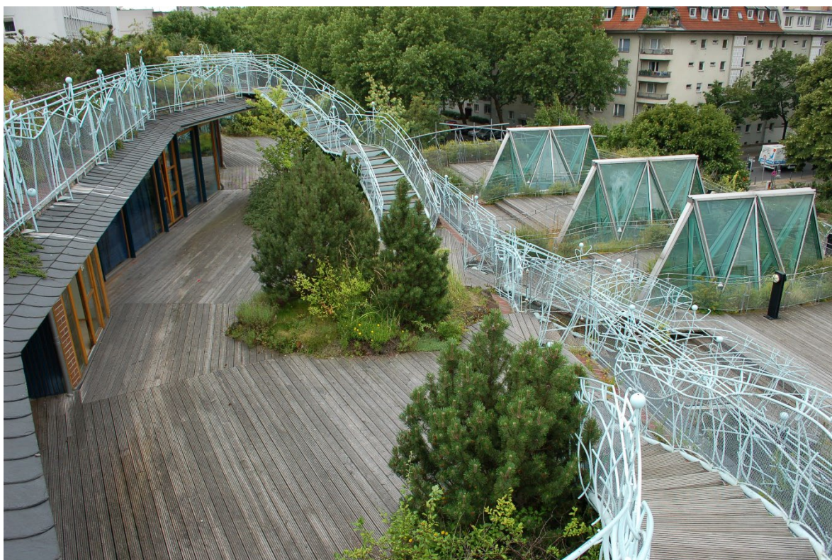
Fig. 7: Elementary school Spreewaldgrundschule in Berlin (Germany), designed by H. Baller. Accessible roof garden.
