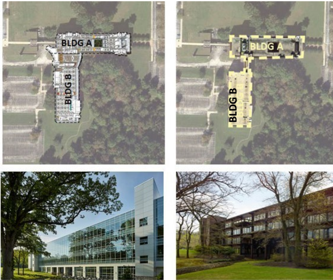
Figure 1. Study Context 1 – A Double Platinum LEED™ All-Glass Office Building.
