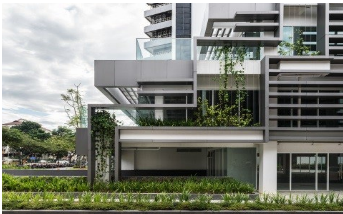
Figure 5: VADS. Sensors integrated into the facade system for irrigation from the rainwater harvesting system.
