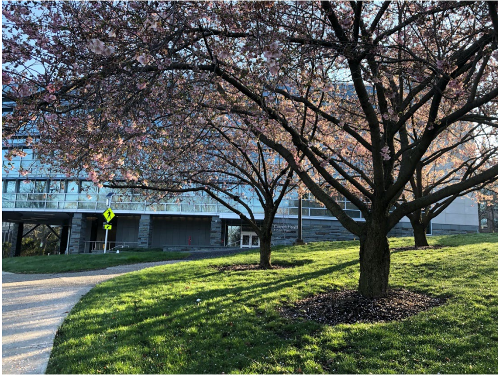
Figure 4: Approach to health building from the south (source: authors).
