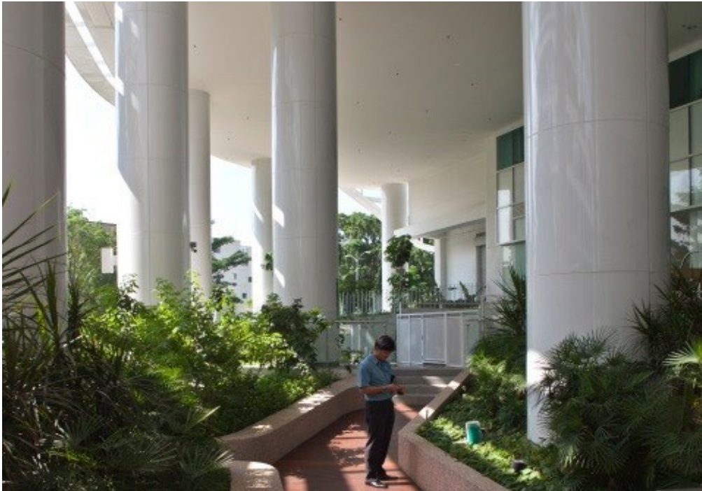
Figure 4: Solaris. A green path between structural columns.
